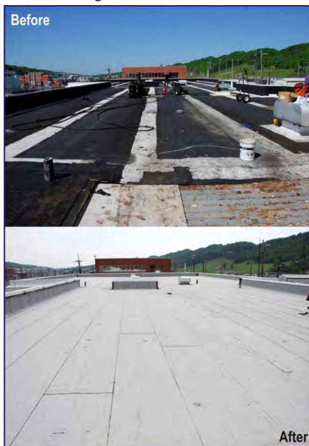
Figure 11-2. Roof repairs on Building 9113 at Y-12. FIRP replace 21,300 square feet of roofing on time and within budget.
